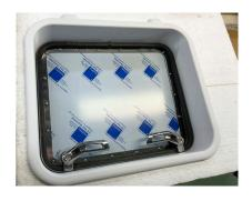
5. Cut the ABS inner frame to the correct depth. Remove the plastic cover on the Velcro pieces and push the composite innerframe in place.
